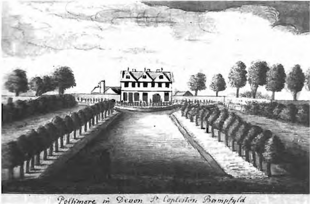
Figure 1. Edmund Prideaux's drawing of the canal front (north-facing) in 1716, inscribed 'Poltimore in Devon Sr Copleston Bampfylde'. Reproduced by kind permission of P. J. N. Prideaux-Brune Esq. from the collection at Prideaux Place.
