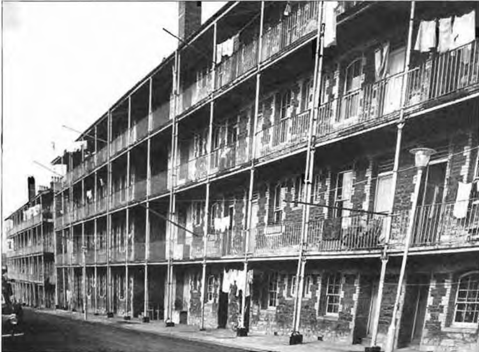
Figure 4: Clare Buildings, Clare Place, Coxside, Plymouth, photographed in 1965 (reproduced by kind permission of the Plymouth and West Devon Record Office, 1479/34).
