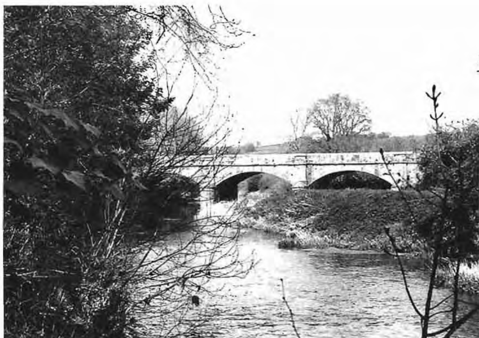
Figure 3: Newnham Bridge, the River Taw (SS 660 174).
