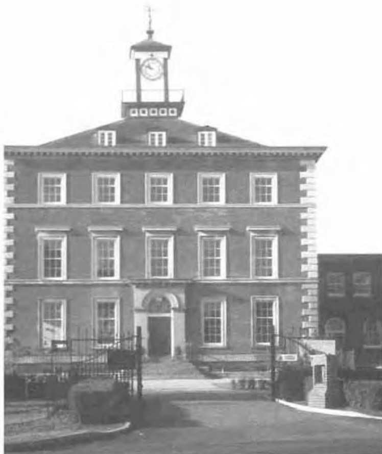
Figure 3: The administrative block.
