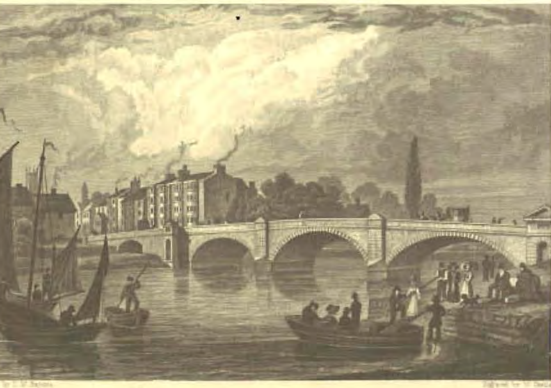
THE NEW BRIDGE, TOTNES, 1810.
