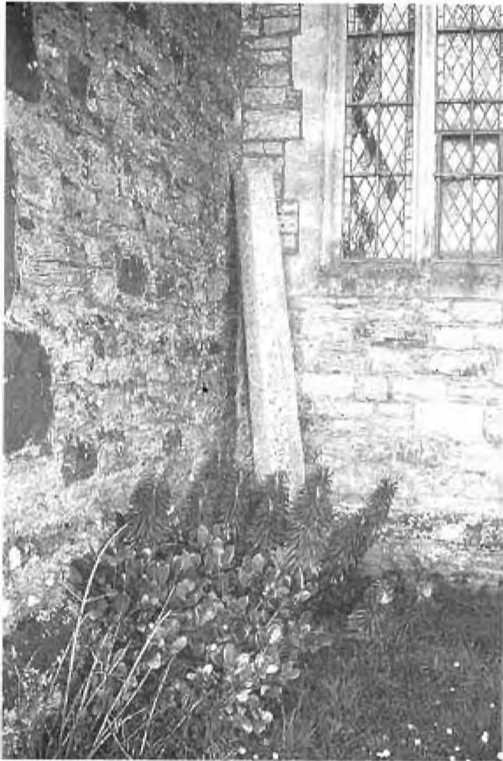
Figure 1: the cross shaft against the wall of the church porch (photo: John Risdon).
