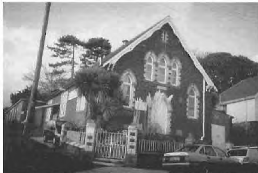
Figure 4: Innerbrook Road Mission Chapel (now the Torbay Olympic Gymnasts' Club).
