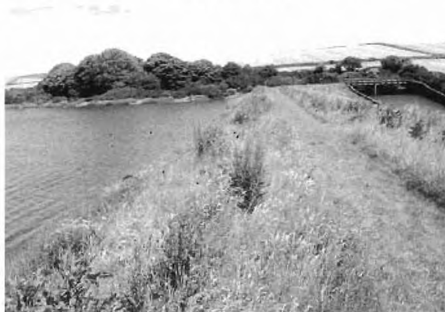
Figure 5: Looking along the dam of Lower Tamar Lake, showing part of the former reservoir of the canal.
