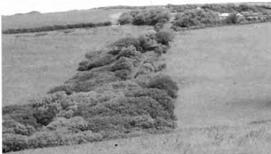
Figure 2: The line of the Hobbacott inclined plane, on which boats were raised 225ft; now much obscured by tree growth, seen from across the valley.
