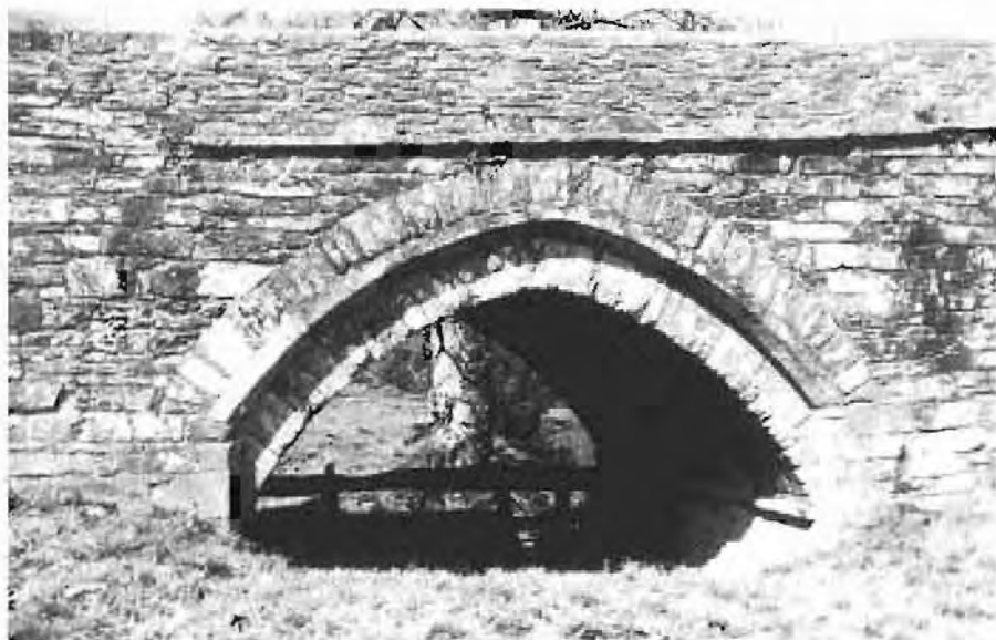
Horse Bridge. Land span on Cornish bank.
