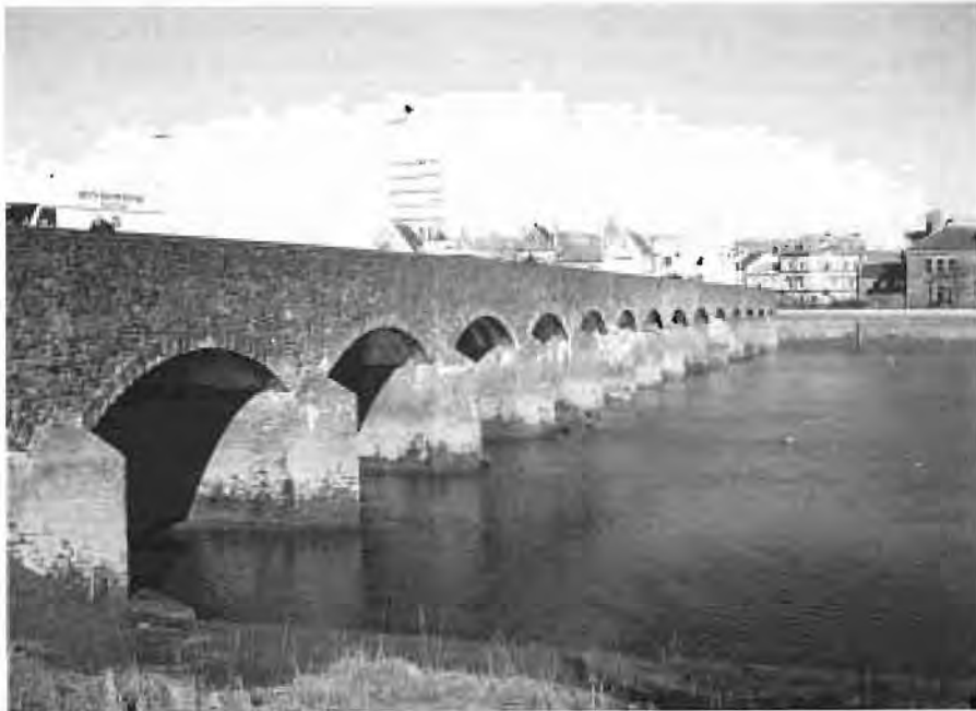
Barnstaple long bridge: upstream face as widened with segmental concrete arches in 1961-1963.
