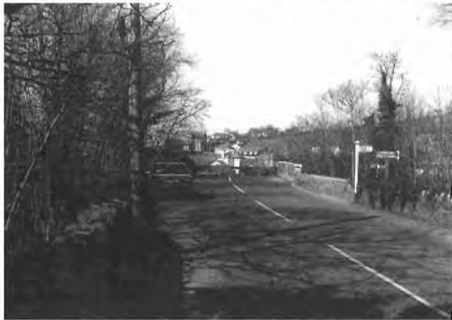
Green's capacious bridge over the River Erme, looking towards Ermington. The smaller structure over the Ludbrook is in front of and beneath the photographer.
