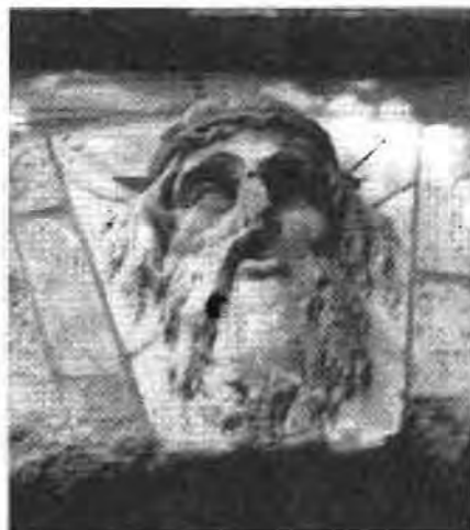
Keystone on southerly face of bridge over Stover Canal
