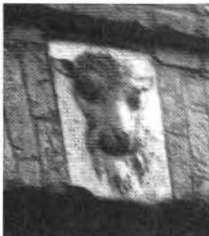
Keystone on northerly face of bridge over Stover Canal
