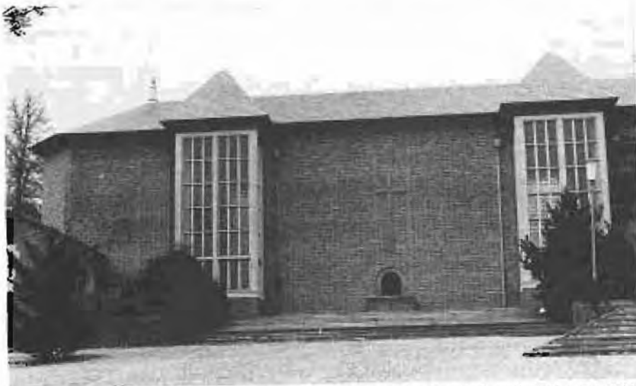
D. Devon has some 25,000 'listed historic buildings'. This listed chapel, dating to 1958, is the 'youngest' one.
