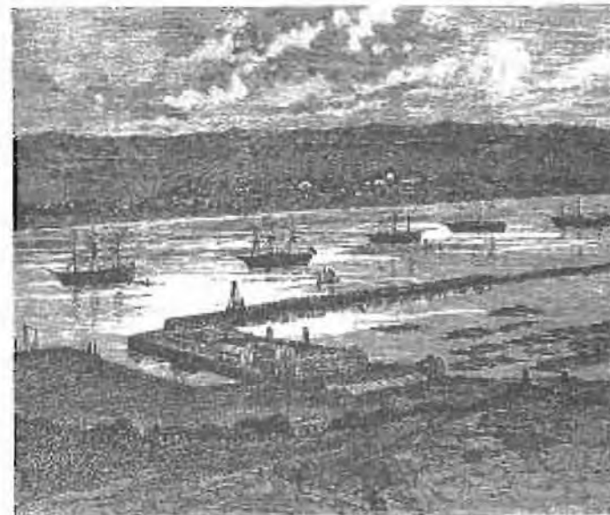
Pile driving at Devonport.
