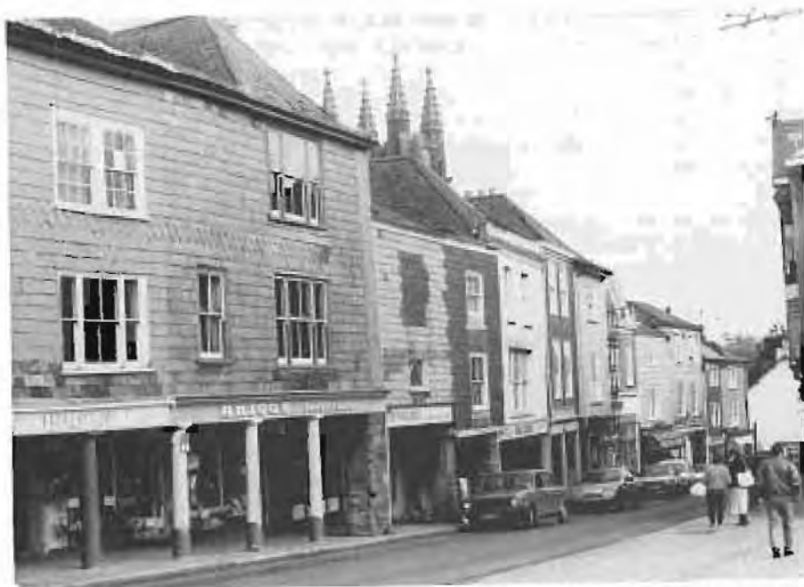
C. To many, this is Devon's finest historic town. A Town Scheme for grant-aiding the repair of historic buildings operates here, and the County Council has undertaken an Enhancement Scheme.
