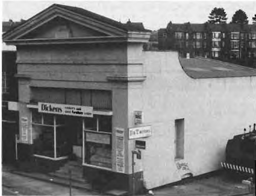
Coldridge's Devon and Exeter Iron, Foundry. Showroom.
