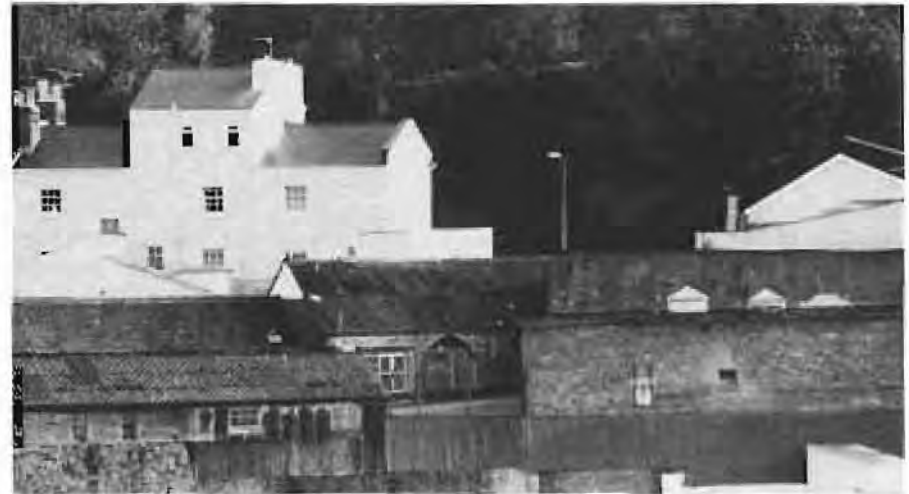
Rear of foundry showing outbuildings at an angle to the showroom.
