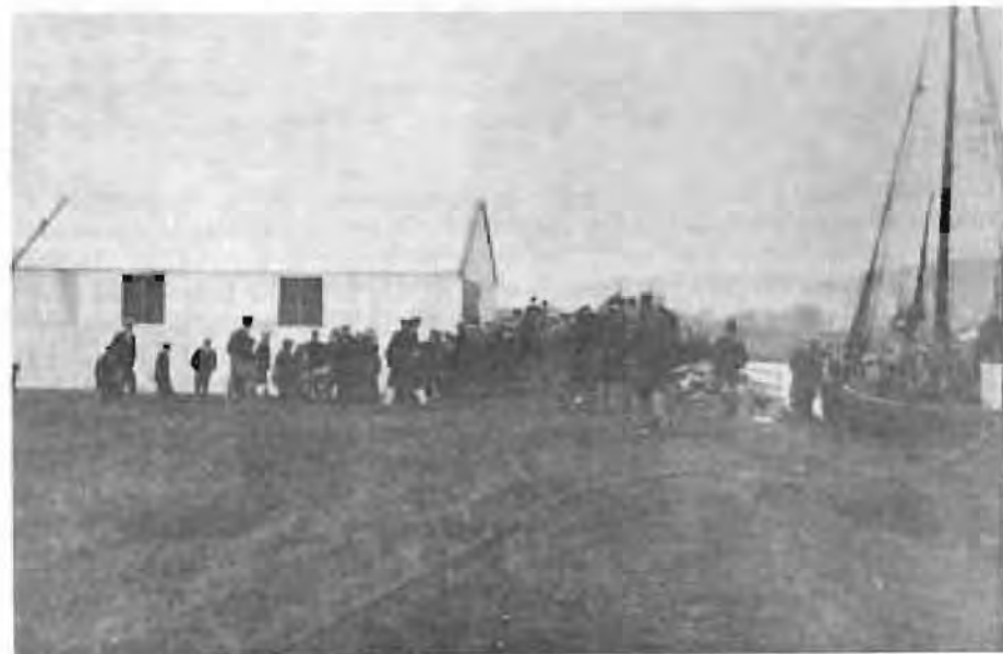
The Crowd at Vellator Quay led by Tom Slee demolishing the buildings.
