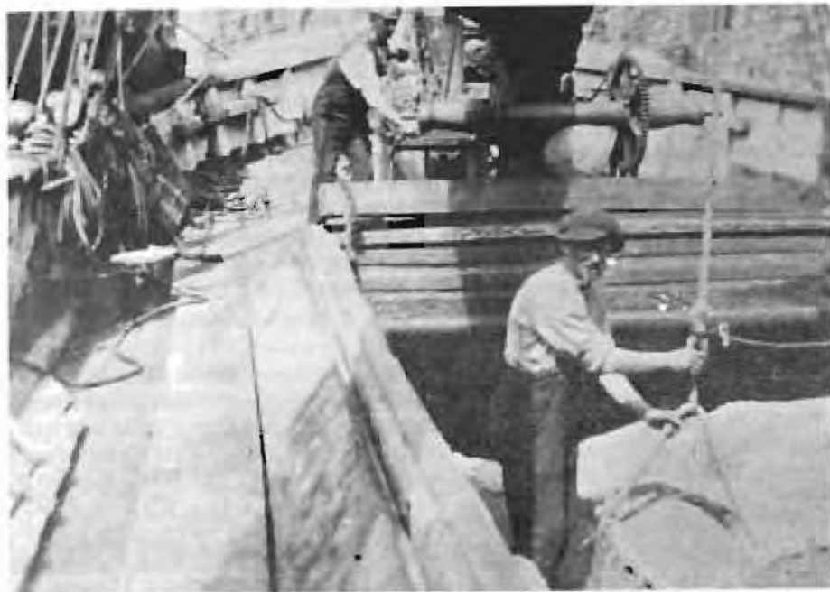
Discharging gravel — Redcliff Wharf, Bristol, 1926. 70 tons in 6 hours. T. Slee filling mawn baskets. Claude Chugg at winch.
