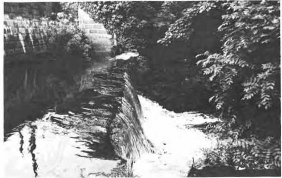
Plate A Present-day view of the weir on the East Okement River which formerly provided the head for the Okehampton hydroelectric station. (Photo by D.G. Tucker)
