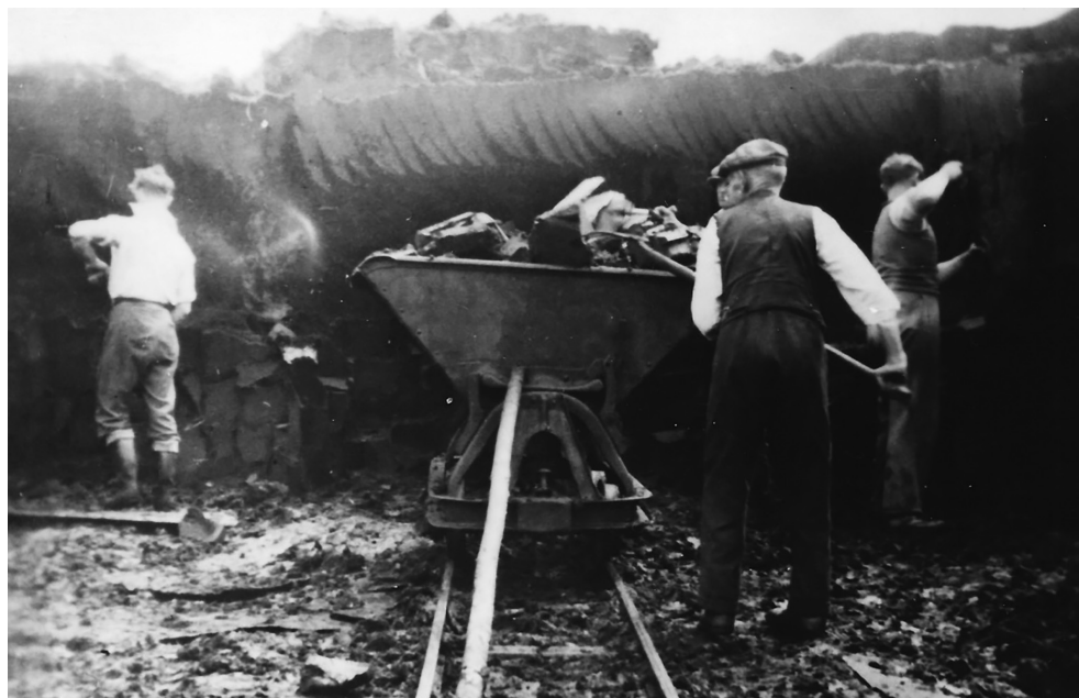
Figure 3. Workers loading peat into a narrow gauge skip wagon. The depth of the workings is readily apparent (photograph © G C Brooks).
