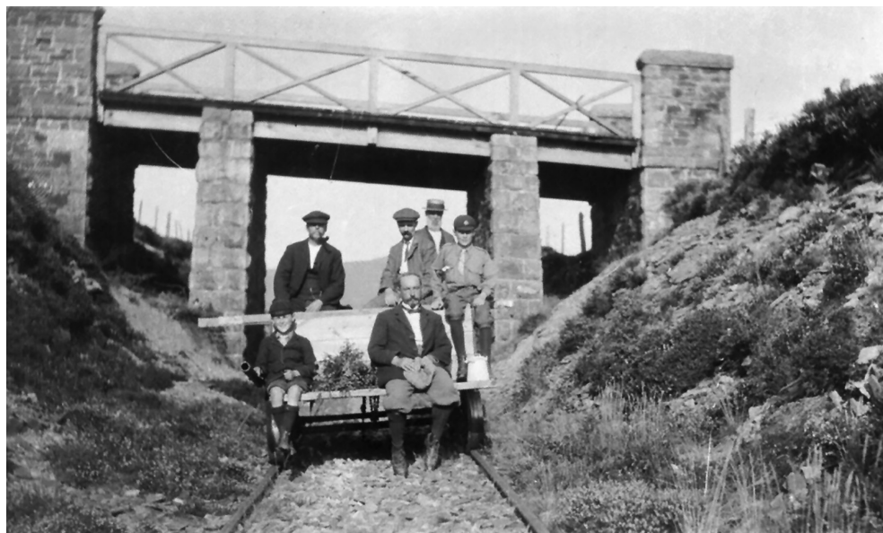
Figure 4. Posed under the only over-bridge on the line (now demolished), this is presumed to be the motorised wagon that the Prince of Wales travelled down the line on (courtesy of Neil Parkhouse).
