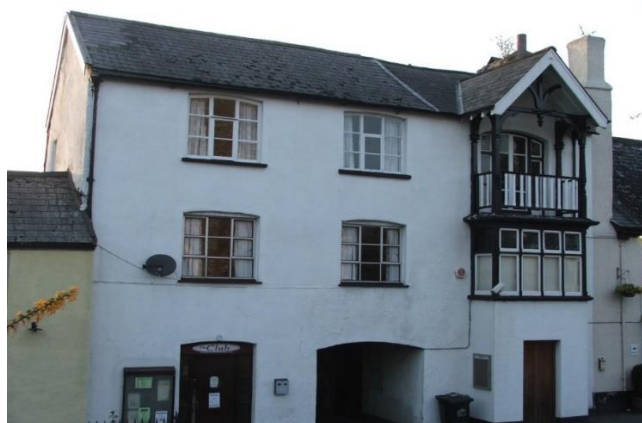
Former National School and workhouse, now the Constitutional Club
