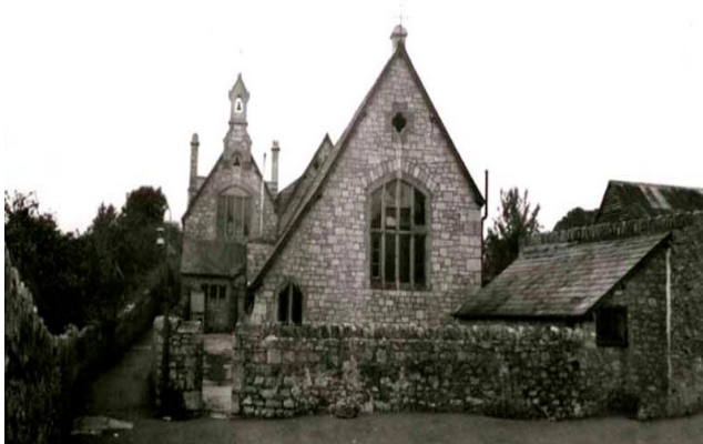
Former National School, now providing a library and Youth Club venue
